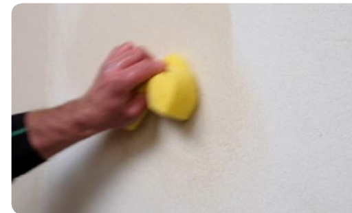
Final phase: wiping the surface (3:40) ▶
