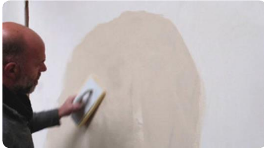
Wiping repaired surface (2:40) ▶
