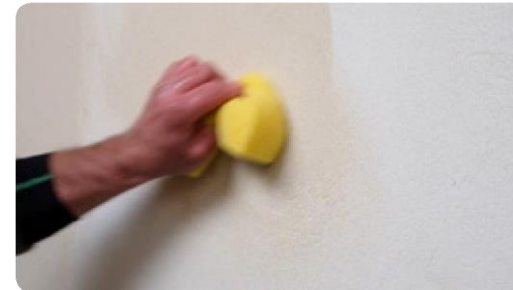
Final phase: wiping the surface (4:00) ▶
