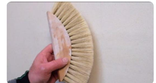
Final phase: brushing the surface (5:00) ▶
