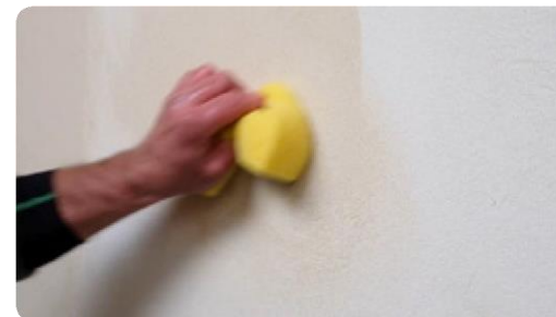
Final phase: wiping the surface (4:45) ▶
