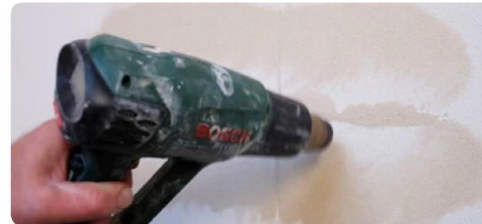
Drying the surface with a heat gun until leather dry (2:50) ▶
