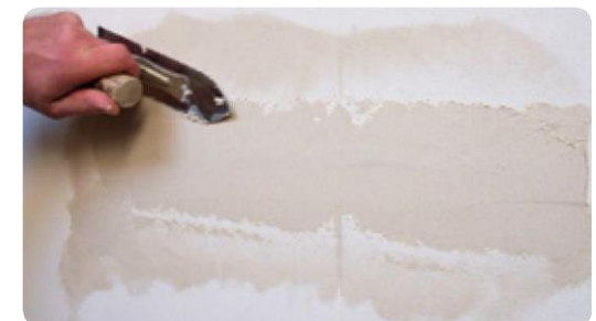
Iron edges for smooth transition (2:30) ▶
