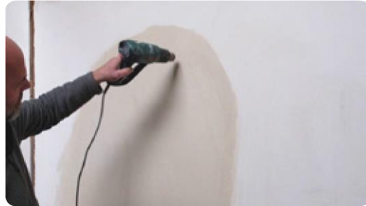
Drying the surface with a heat gun (3:30) ▶
