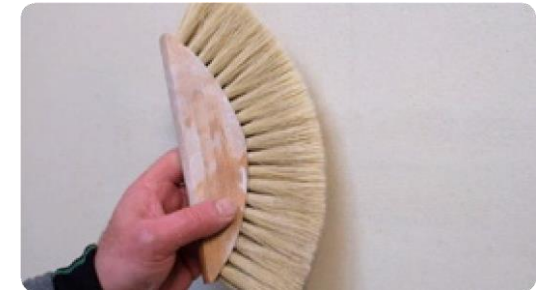
Final phase: brushing the surface (4:30) ▶
