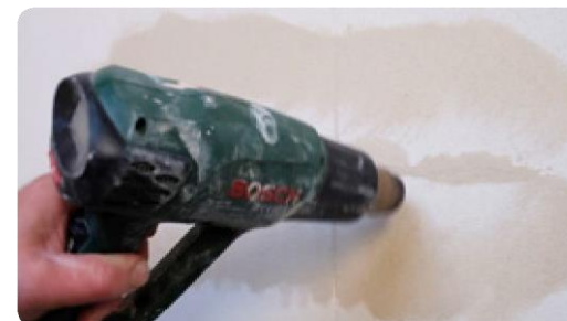
Drying the surface with a heat gun (2:00) ▶
