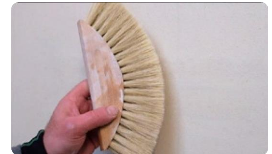
Final phase: brushing the surface (4:15) ▶
