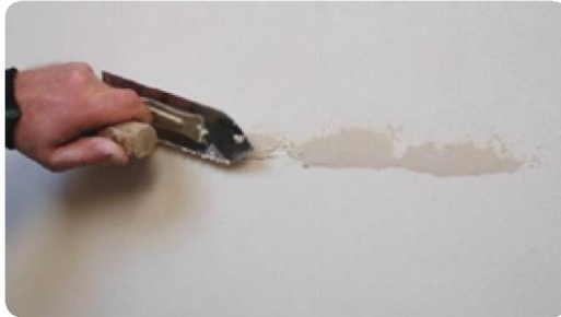
Filling scratches (1:00) ▶
