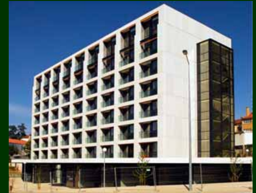
Studio Residence - Coimbra
